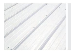
By reflecting sunlight, the white R NOVA PLUS liquid system reduces the roofing system temperature and increases its service life. Furthermore, it contributes to obtaining the LEED SS Credit 7.2: Sustainable Sites – Heat Island Effect: Roof.
